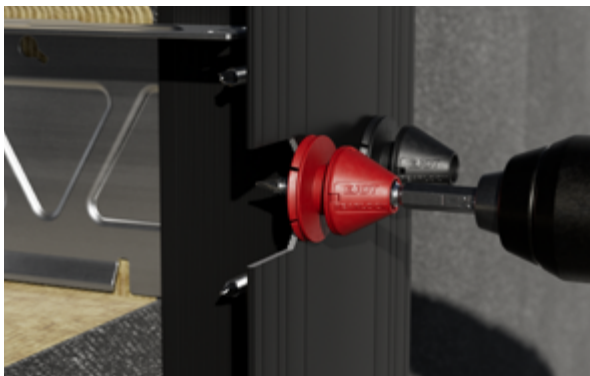
The screw is screwed in up to the stop collar. It ensures a precise installation depth, creates a defined clamping range and guarantees reliable perpendicular alignment of the screw.
